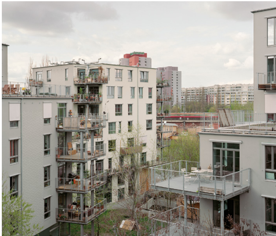
Public access at Spreefeld Berlin is created with permeable solitary blocks that extend through to the Spree river. Image: Andrea Kroth
